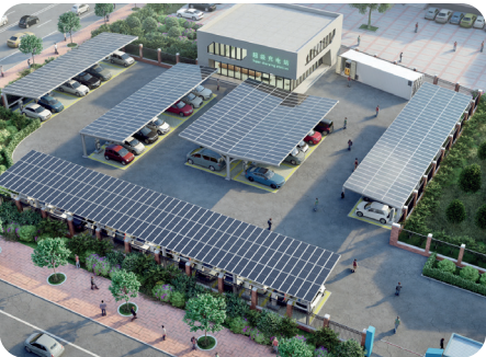
PV Charging Carport With Storage
