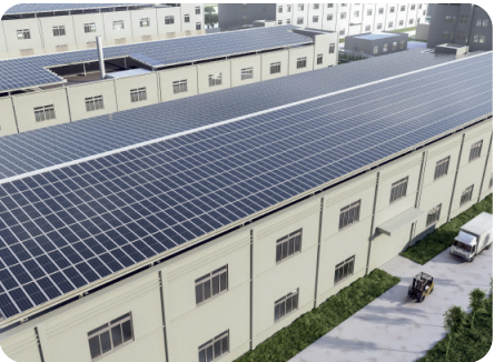
Flat-to-pitched Roof Conversion
